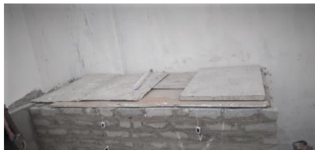
Fig 4. Two rooms with temperature measuring devices source: self
